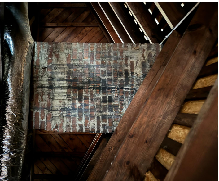
View in attic
